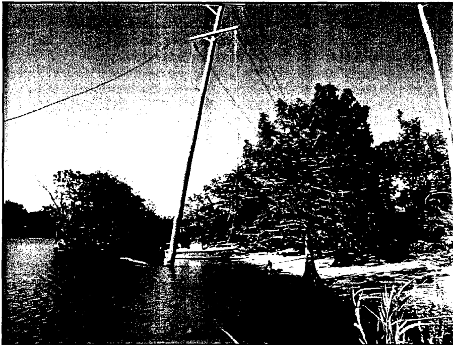
Figure 6-17. HNC-7 on the east bank of the Houma Navigation Canal. View to the northeast. Date: 10/22/03.
